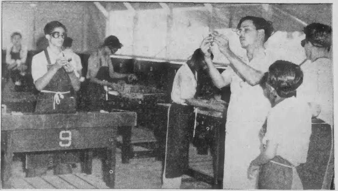
Rafael Wever, instructor in the machine shop, demonstrates the correct method of checking the angles of a piece of metal to see that they are perfectly square. Working with a round piece of metal, the boys file it down into a square shape. Then, with a try-square, they check each side to see that the object is perfectly square.
